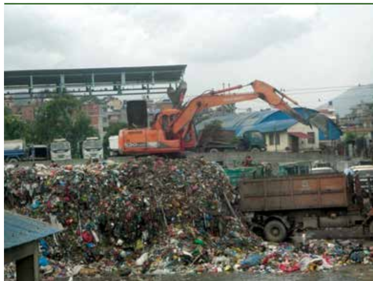
Photograph 4: Waste being Loaded for Transfer to Landfill from Teku
